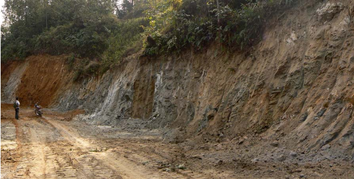
Section of the soil structure near a newly constructed road near Kajeri in the Kaski District of Nepal. Many different shades of colours can be easily identified, which indicates many different types of soil.
